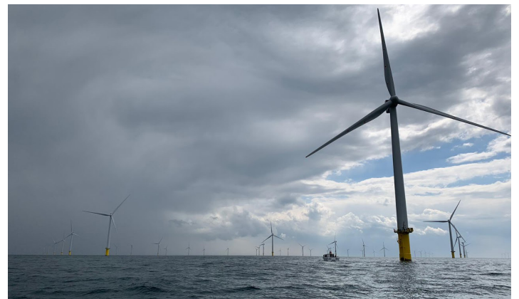
Scotland Windfarm Trip
