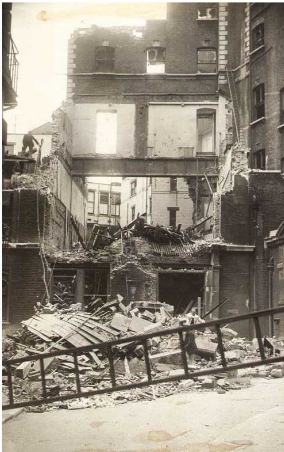
Bomb damage to the Medical Lecture Theatre, 1940
